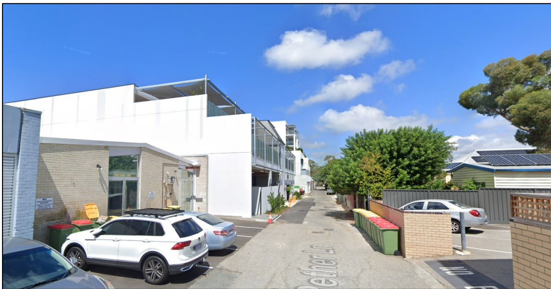
Figure 6 — As-Constructed Shade Structure (View from Pether Lane – Image 2)
