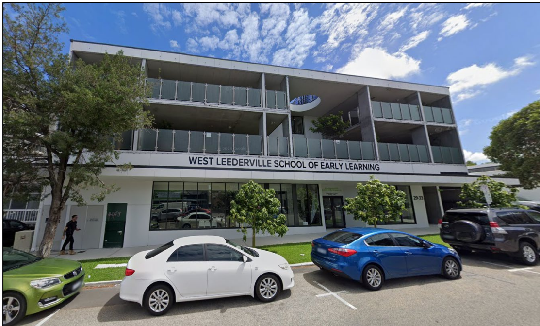
Figure 8 — As-Constructed Northwood Street Elevation (Google Street View)
