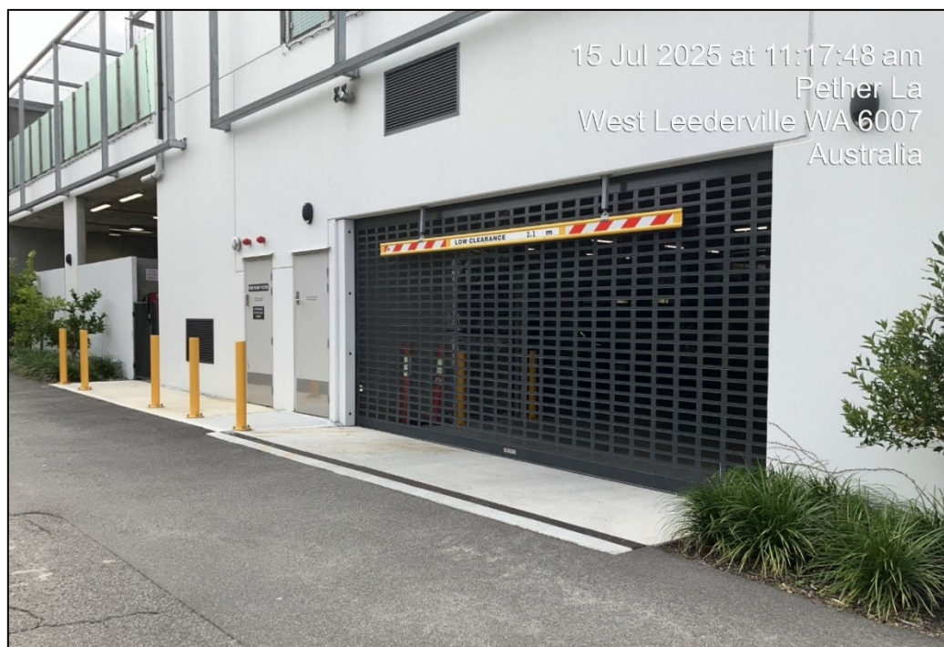
Figure 11 — As-Constructed Perforated Garage Door (Western Elevation)
