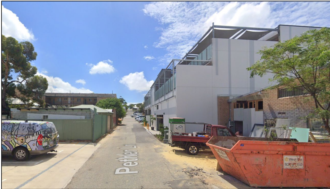
Figure 5 — As-Constructed Shade Structure (View from Pether Lane – Image 1)
