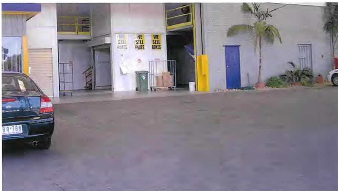
Photograph 2-6: Loading area located adjacent to service lift
