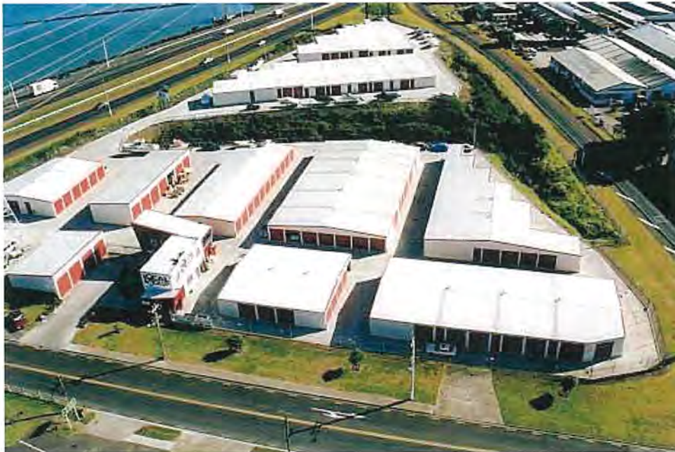
Figure 1: Ranch Style Self Storage Facility
