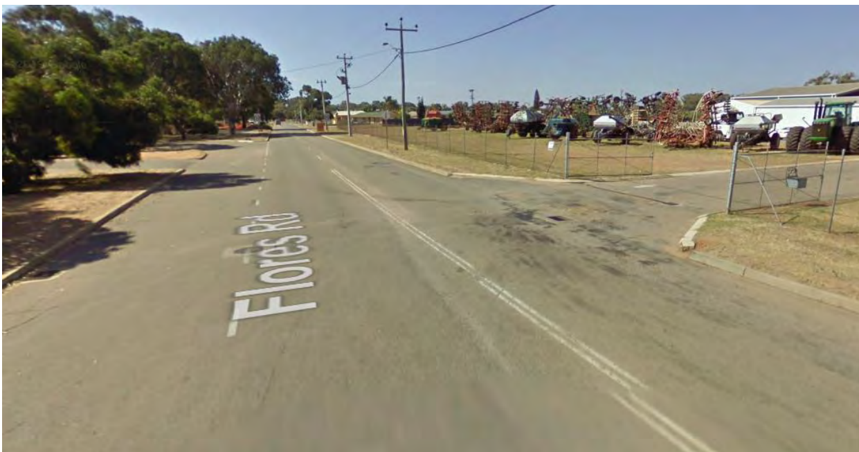
Figure 2. Northbound view along Flores Road, adjacent to the subject site
