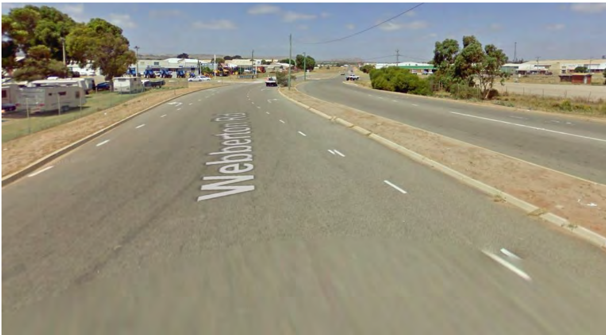
Figure 3. Eastbound view along Webberton Road, adjacent to the subject site
