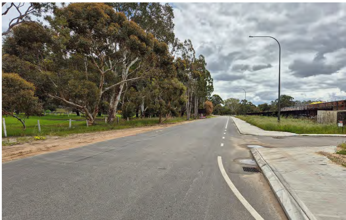
Figure 4: Westbound view along Henley Street in the vicinity of school site
