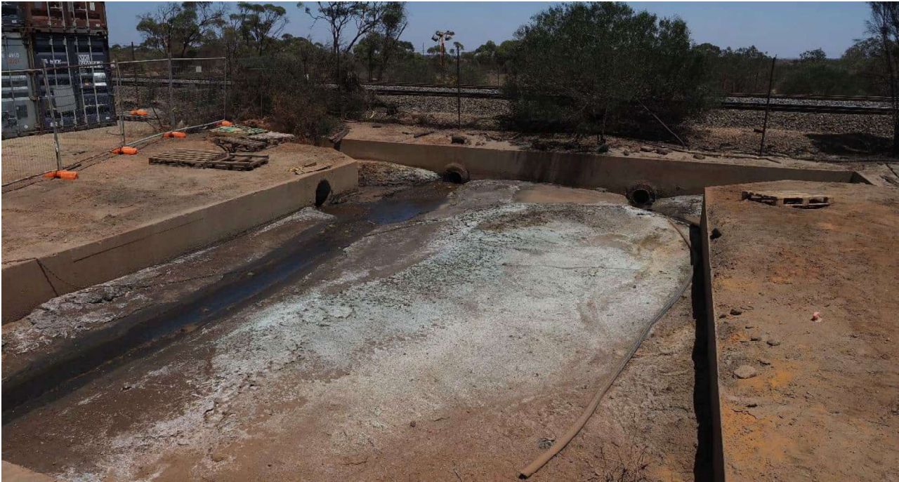
Plate 1: Drainage pit upstream of the railway
