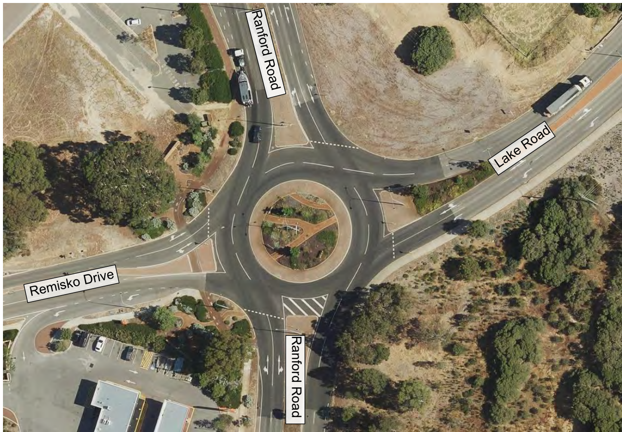
Figure 2-4 Ranford Rd / Remisko Dr / Lake Rd Intersection
